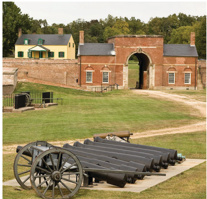
Fort Washington, Maryland
