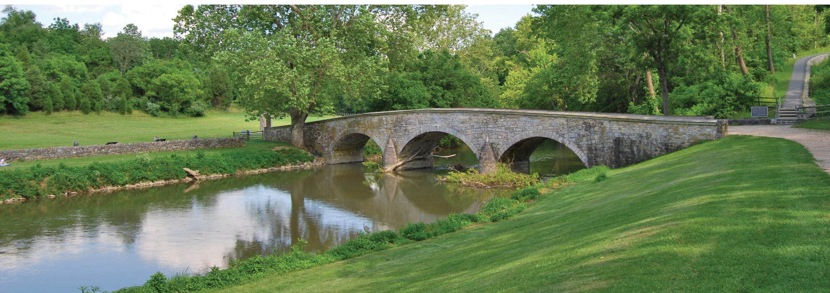
Burnside Bridge at Antietam National Battlefield, Sharpsburg, Maryland
