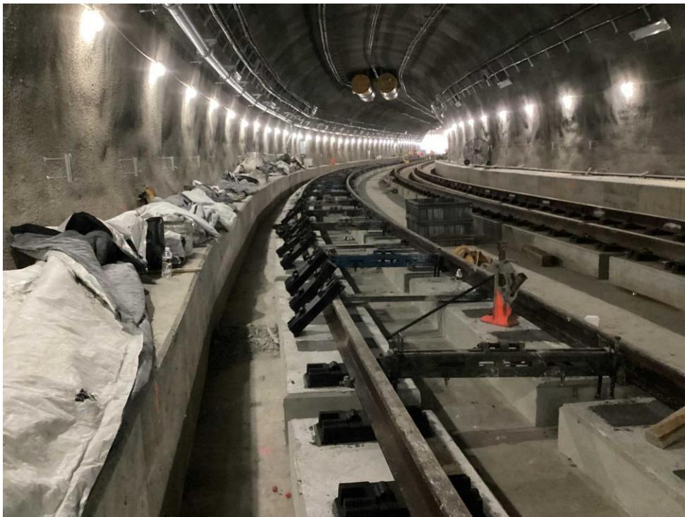
Direct Fixation Track – Site view of direct fixation tracks #1 and #2 work progress from the Tunnel towards Arliss Street (11.04.25)
