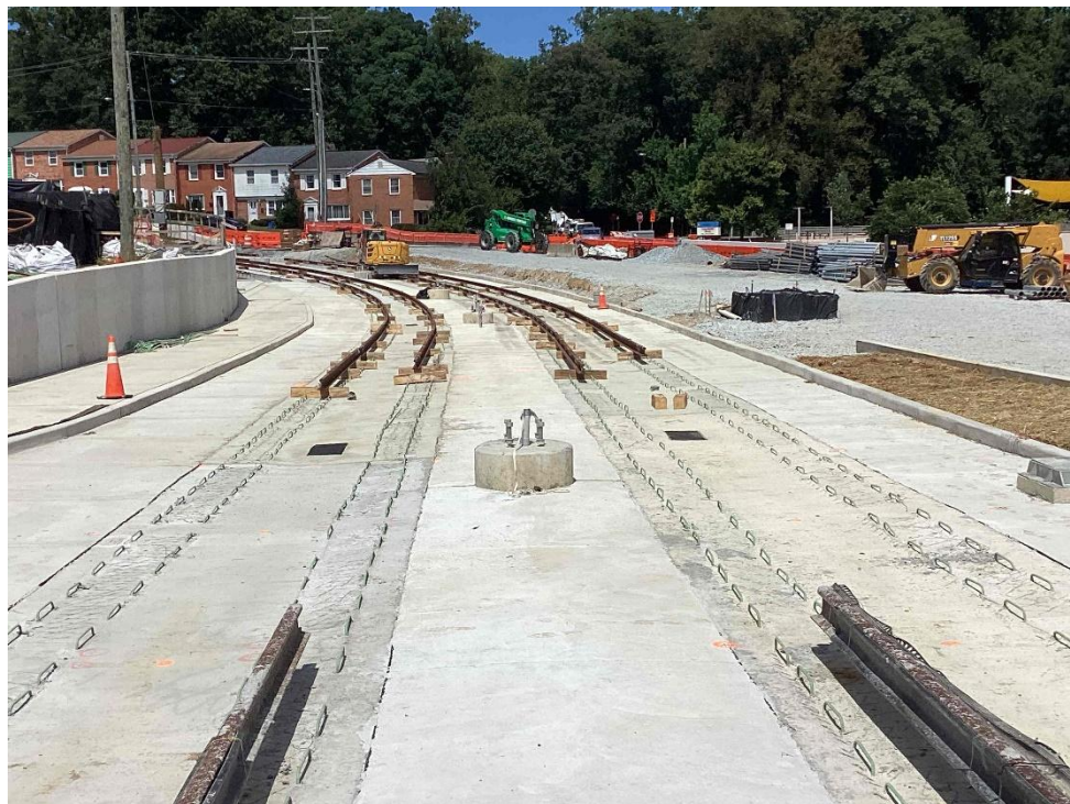
Direct Fixation Track – Site view of direct fixation tracks #1 and #2 work progress from the Tunnel towards Arliss Street (08.28.25)
