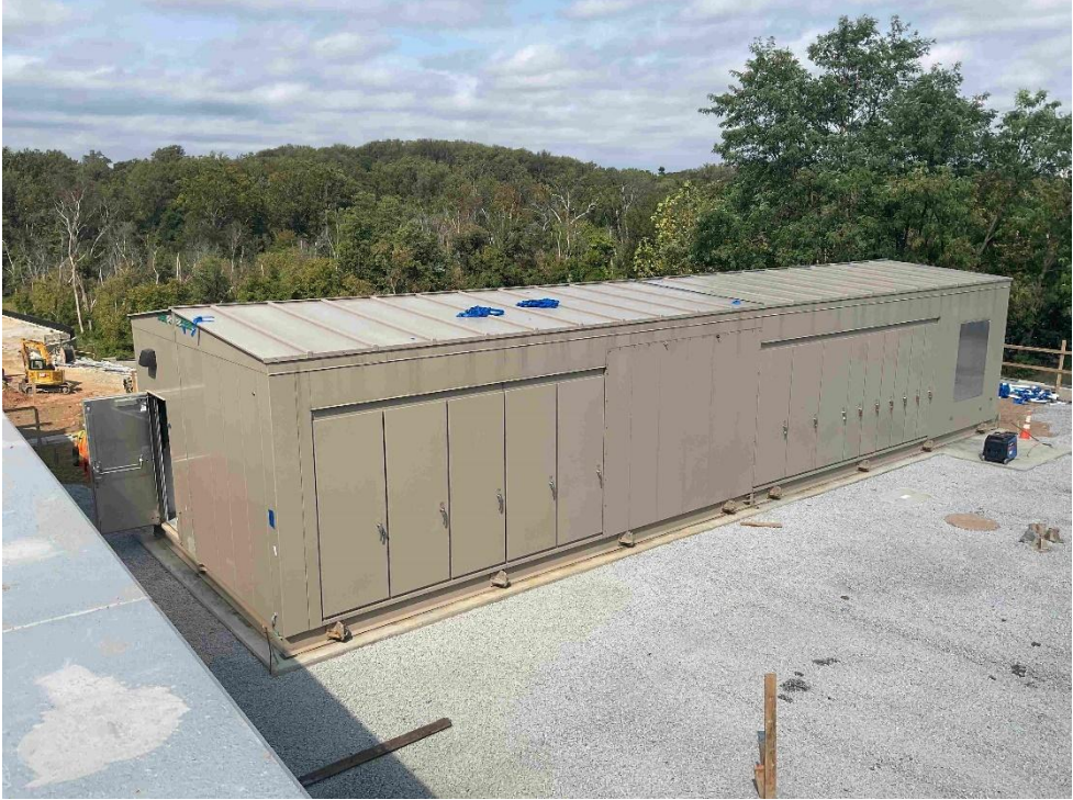
Lyttonsville Yard - Site view of traction power substation TPSS-Q2 set on concrete pad as of 09.22.25.
