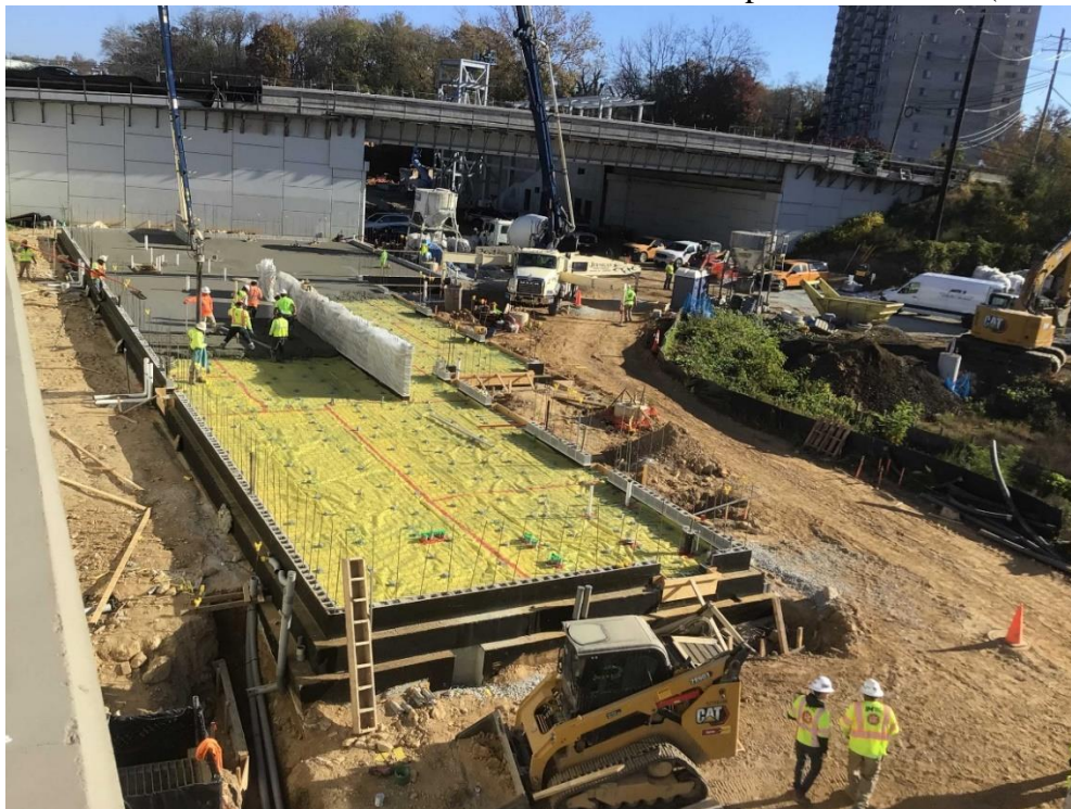
Lyttonsville OMF - Site view of the Foundation concrete placement work. (11.06.24)
