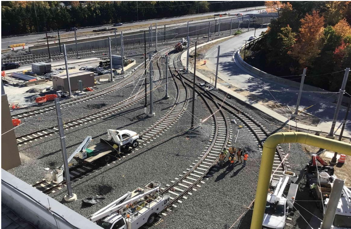
Site View of Glenridge Yard looking East at the ballast track and OCS work. (10.25)
