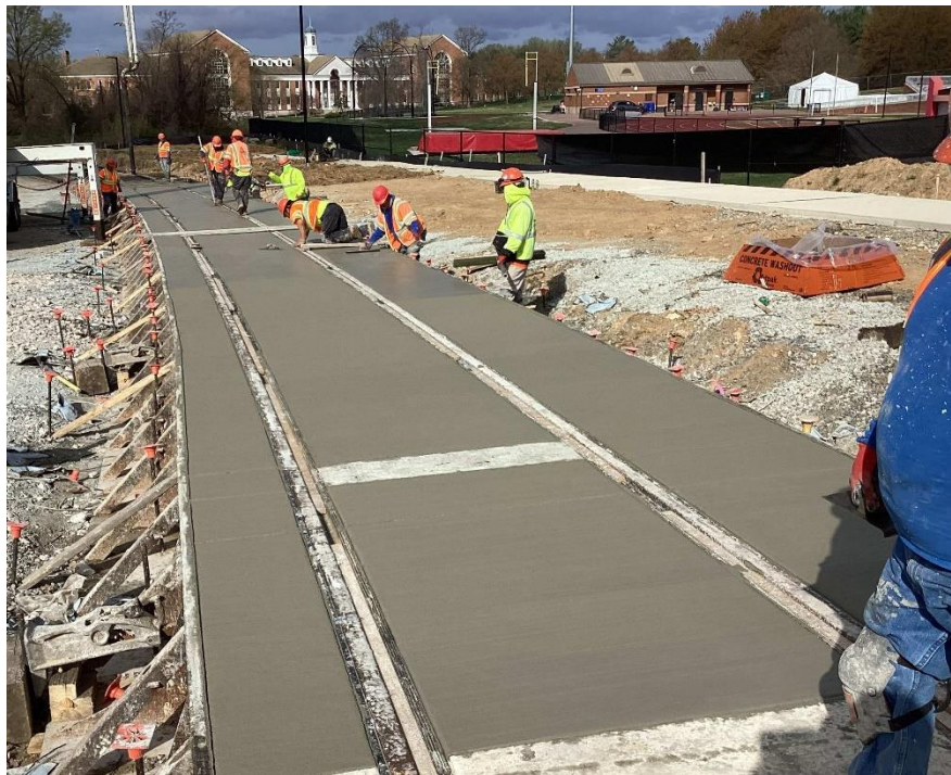
Embedded track #2 concrete placement on Campus Drive. (01.17.25)
