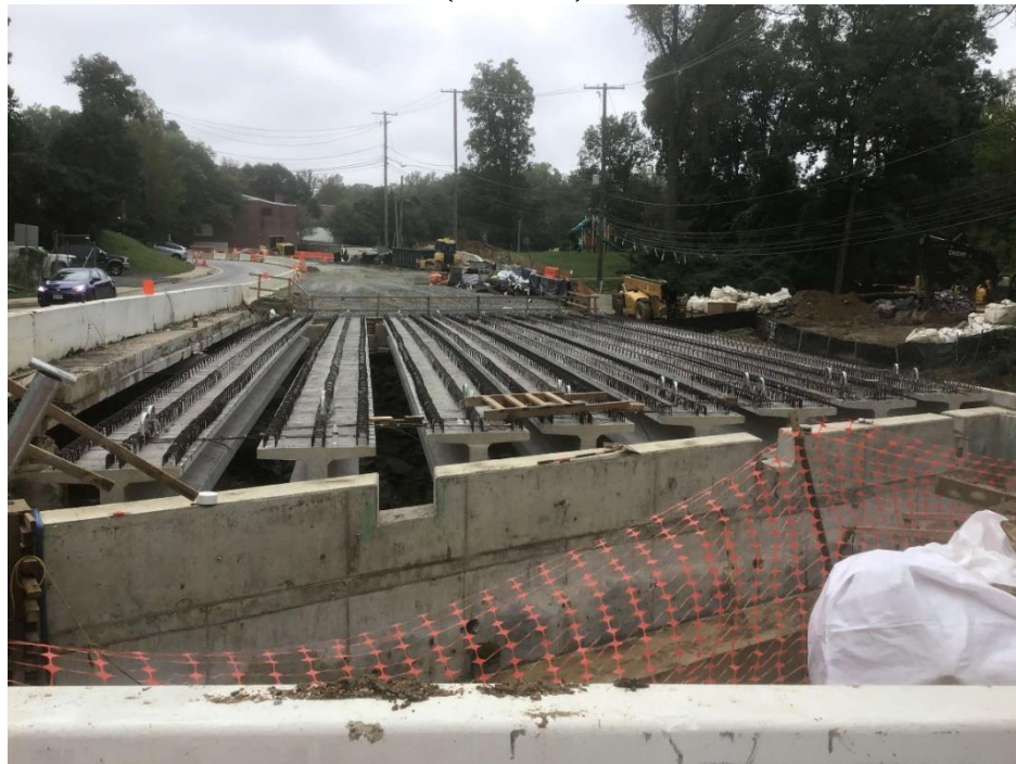
Wayne Ave Bridge – Site view of the completed girders. (09.30.24)
