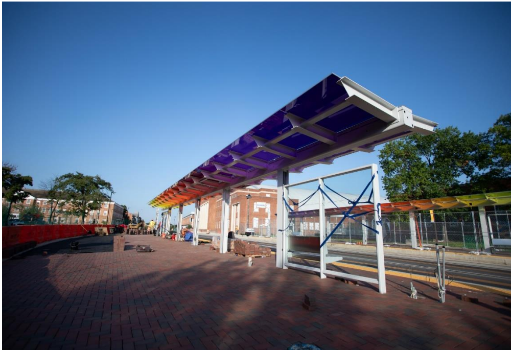
Ground-level view of Campus Drive-UMD station.
