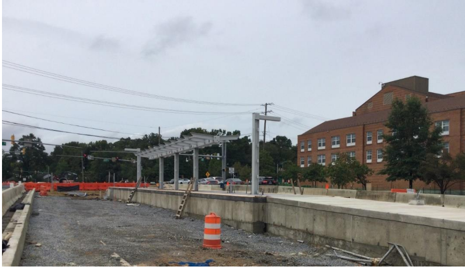
Segment 6 (Adelphi Road to College Park): Adelphi Road-UMGC-UMD Station Platform Canopy and Column progress. (09.23.24)
