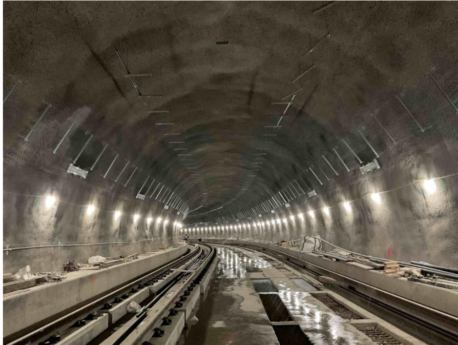
Segment 4 (Manchester Road to Arliss Street / Plymouth Tunnel): Plymouth Tunnel – Site view of the tunnel ceiling rack and conduit work progress. (09.25.24)
