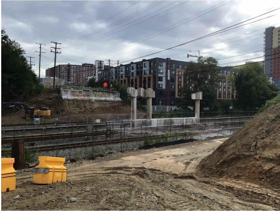
Segment 3 (Spring Street to Manchester Road): Spring Street Bridge Site view of the demolition of existing bridge. (09.19.24)
