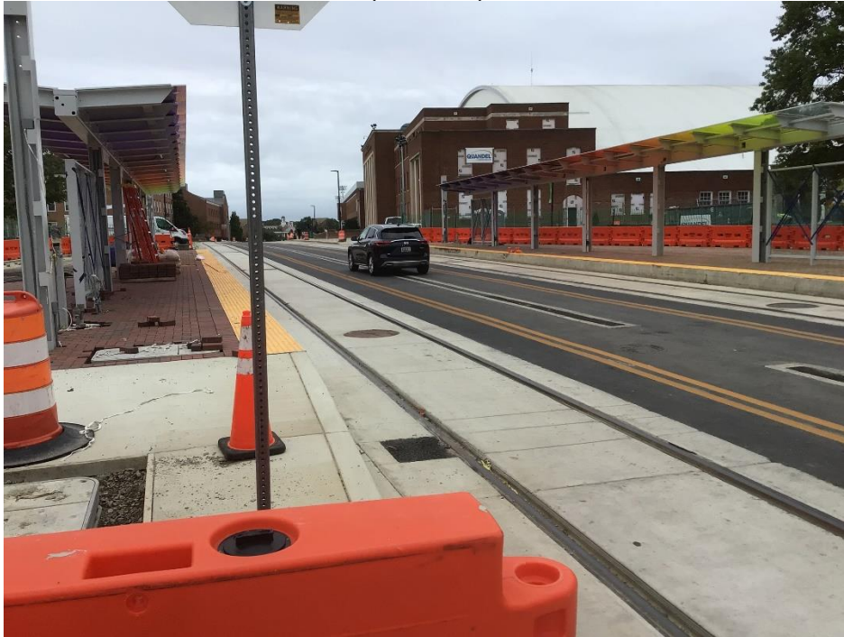
Campus Drive-UMD Station Platform Canopy and pavers installation work progress. (09.23.24)
