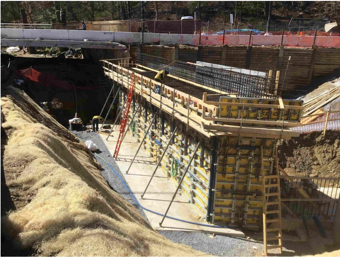
Segment 4: Manchester Place Station – Zone A site view of work progress for the cut & cover box entrance on Wayne Avenue. (03.14.24)
