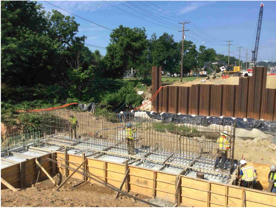
Segment 5 –S27 NW Branch Bridge Abutment at University Blvd. (07/13/23)
