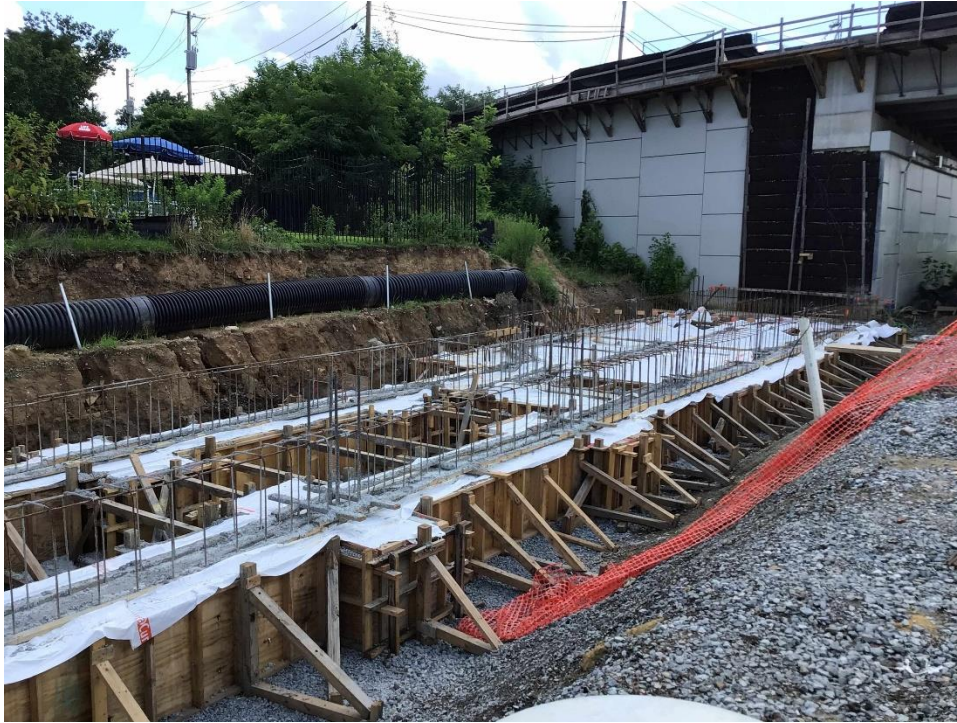
Segment 2 – Core Foundation Concrete under cure at Lyttonsville Station (07/21/23)
