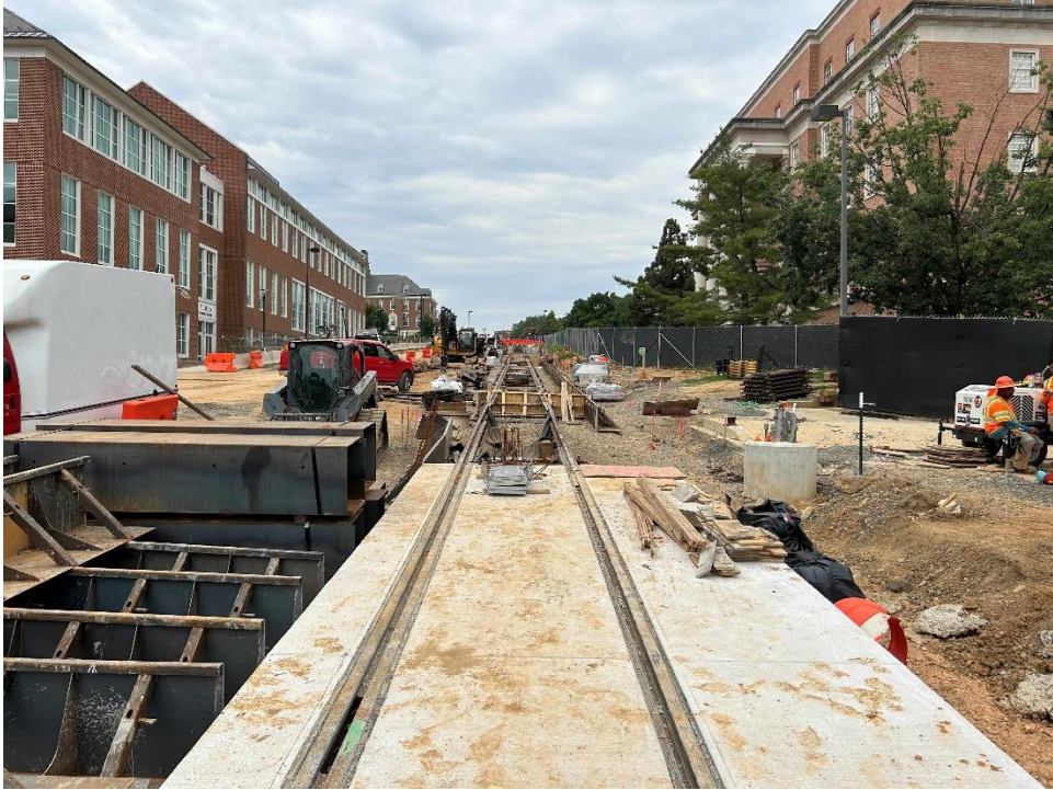
Segment 6 – Embedded Track Installation at Campus Dr.-UMD Station (07/27/23)
