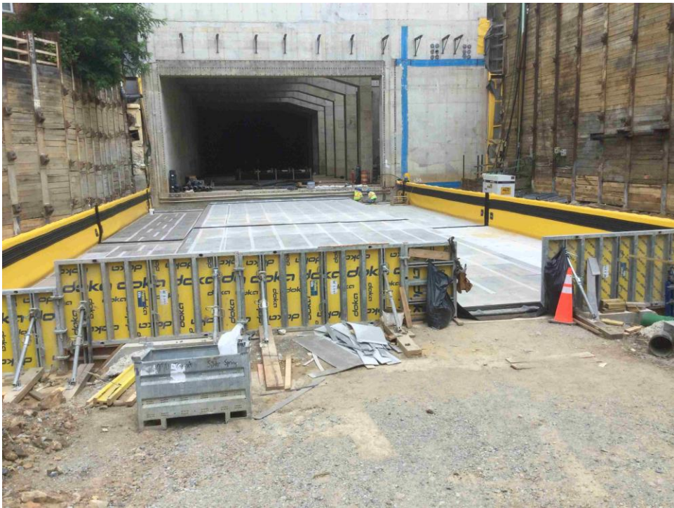
Segment 4 – Mud Mat Cement Boards Install Zone A at Manchester Place (07/14/23)
