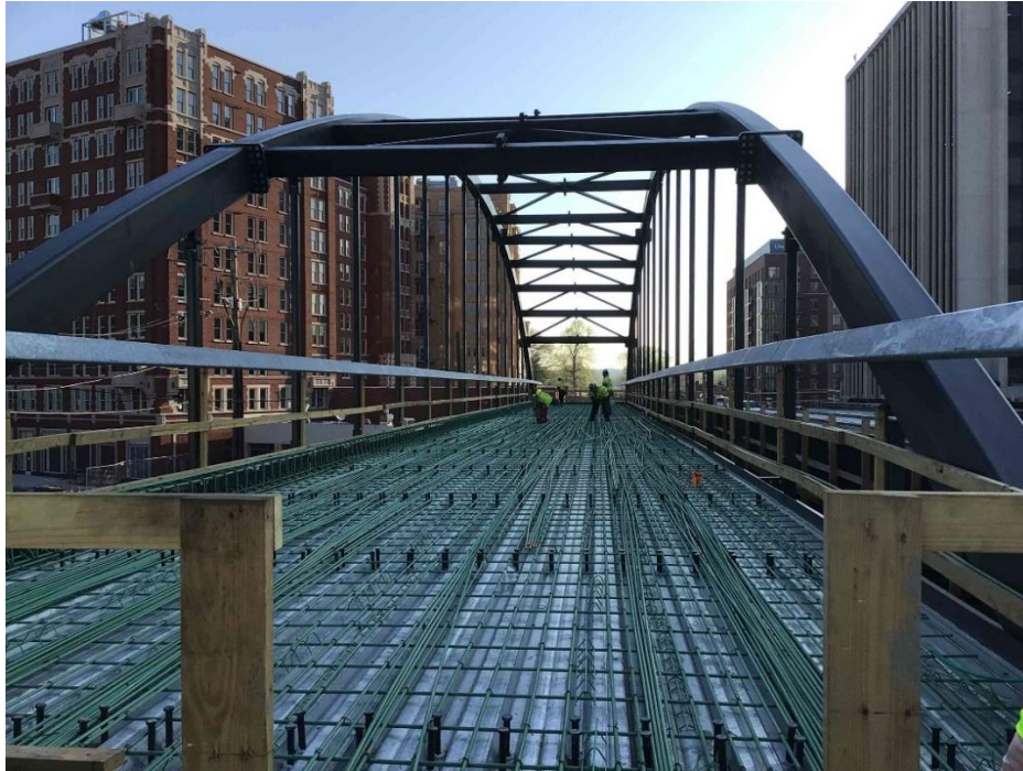
Segment 2 – Structure S07 Pedestrian Bridge Deck Rebar at Connecticut Ave. (04/05/23)
