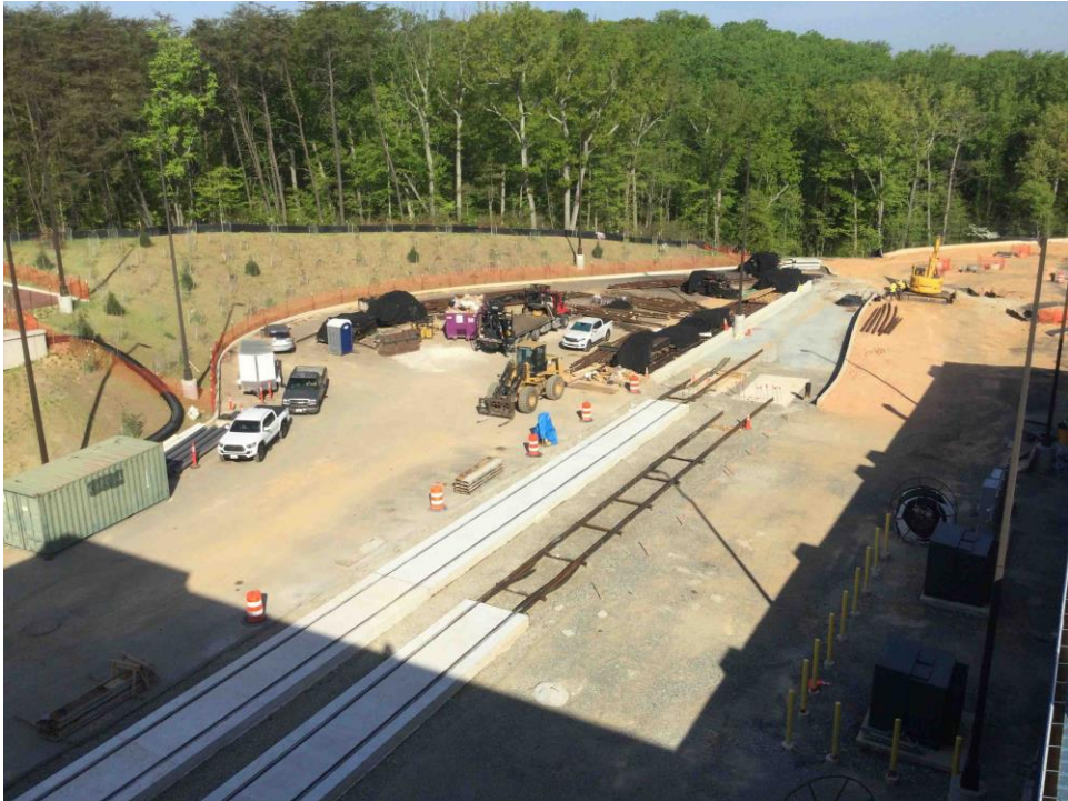
Segment 8 – Roof View looking West of MOW Track Installation at Glenridge (04/19/23)
