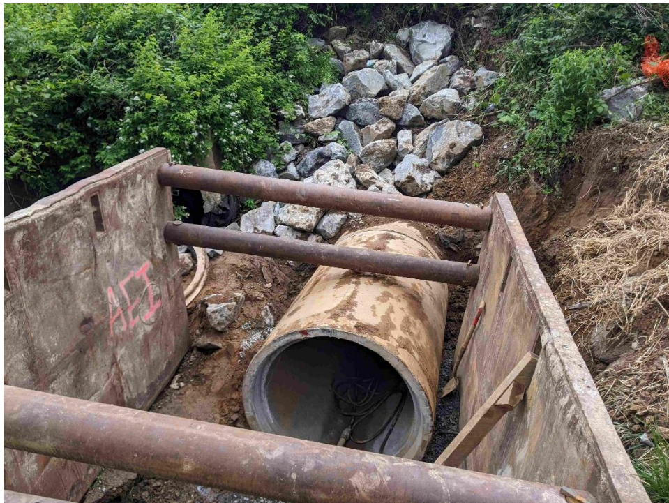
Segment 5 –RCP Installed for Fish Passage at Long Branch Culvert (05/09/23)
