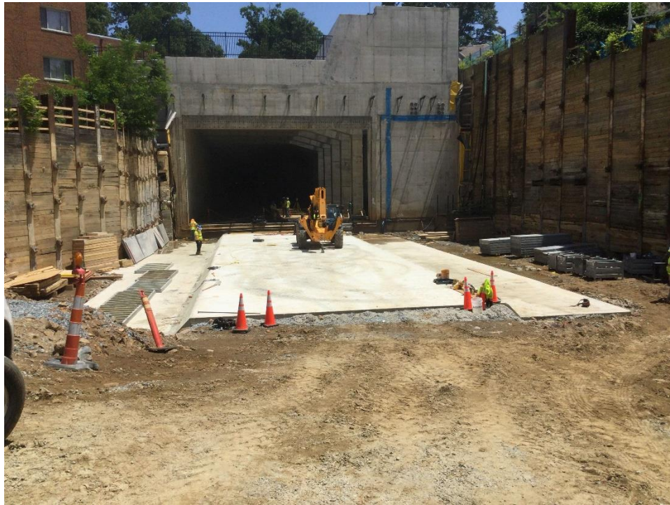
Segment 4 – Mud Mat Concrete Placed at Manchester Place (05/19/23)
