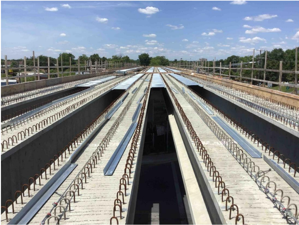
Segment 7 – Structure S29 LRT Bridge over Kenilworth Ave. Deck Pan Installation (05/29/23)
