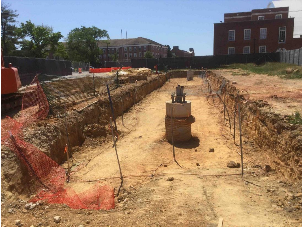
Segment 6 – Ground Rod Installation at Campus Dr.-UMD Station (05/25/23)
