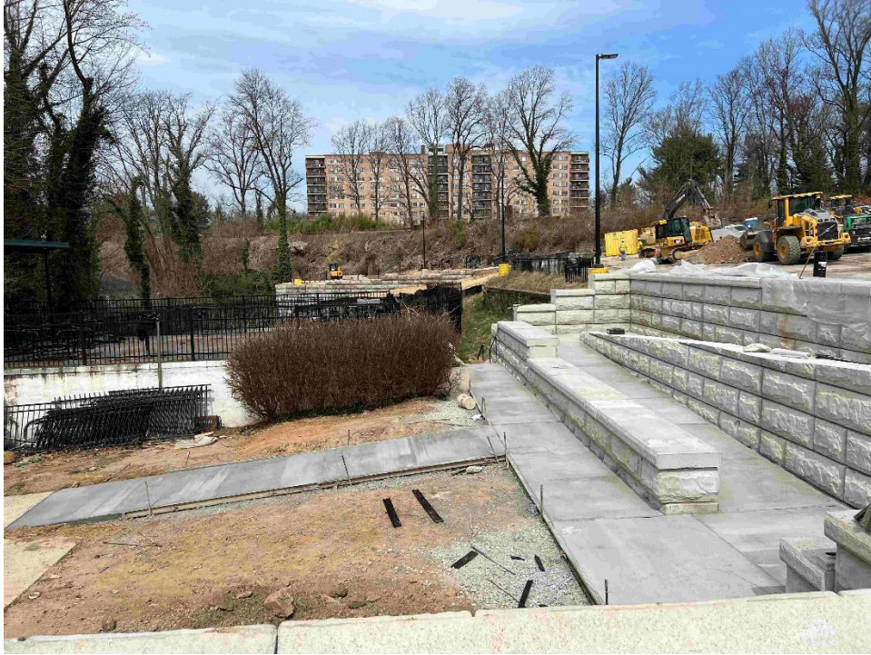
Segment 3 – Sidewalk Concrete Placed at Bradford Place Apartments (03/22/23)
