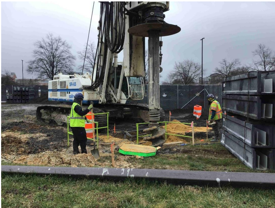
Segment 6 – Catenary (OCS) Foundation Drilling on UMD Campus (03/13/23)
