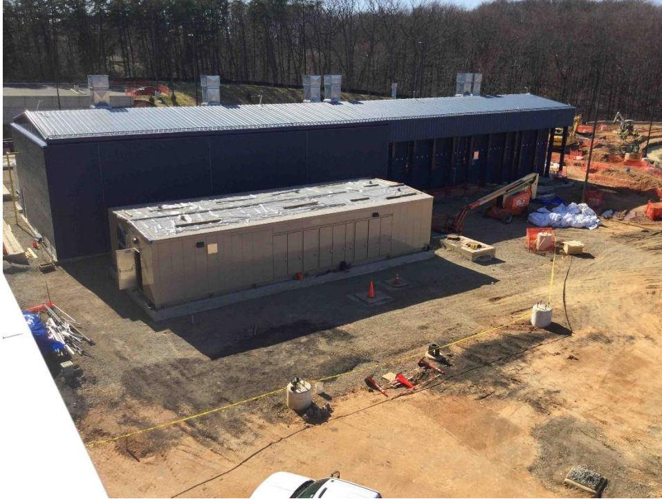
Segment 7 – Substation TPSS-QYG Set-in-Place at Glenridge O&M Facility (03/09/23)
