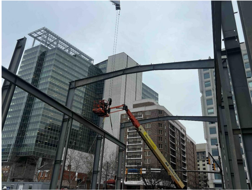
Segment 1 – Gantry Shed Installation at Bethesda Metro South Entrance (03/02/23)
