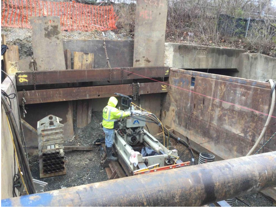
Segment 5 – Directional Bore Drilling for Fish Passage at Long Branch Culvert (03/10/23)
