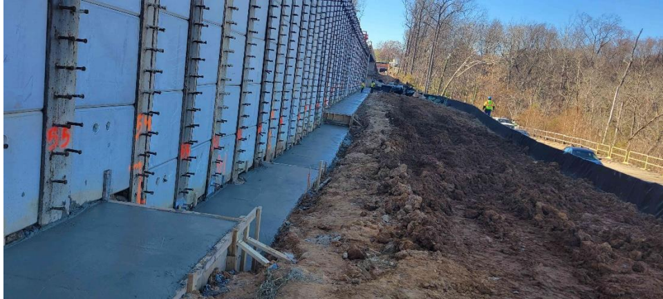
Segment 1 – Concrete Placement for Wall 1-067 near Rock Creek (11/21/22)
