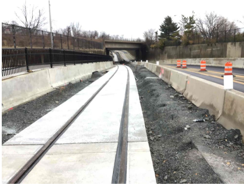
Segment 6 – Embedded Track Construction near College Park Metro (1/3/23)
