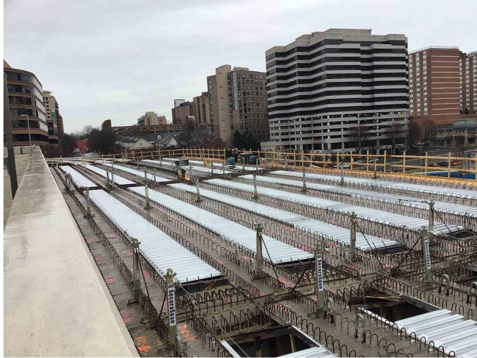
Segment 3 – Deck Formwork for Silver Spring Transit Center Station (1/17/23)
