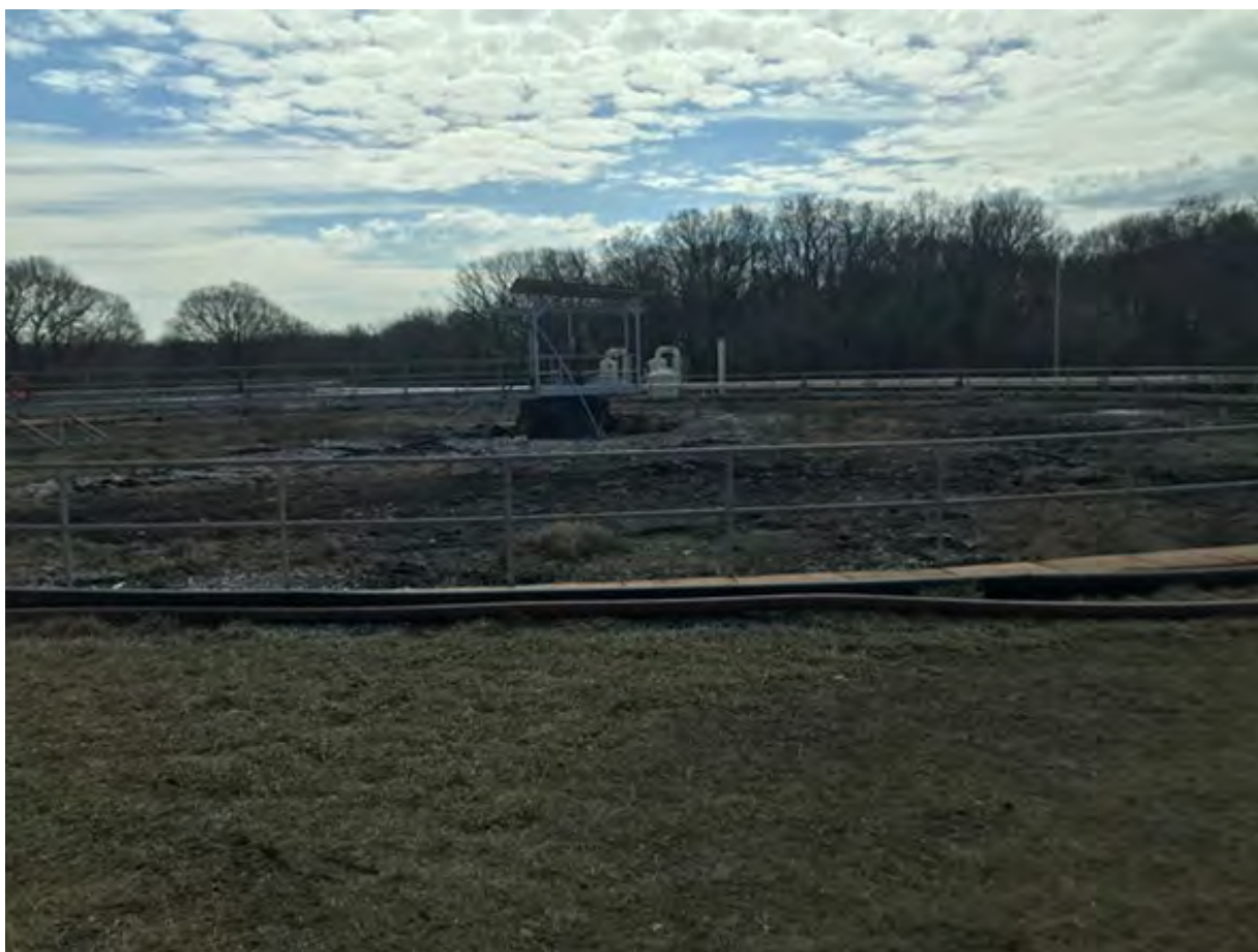
Figure 4 - Back River WWTP – Example of a Primary Clarifier (PST) Filled with Accumulated Solids, March 2022
