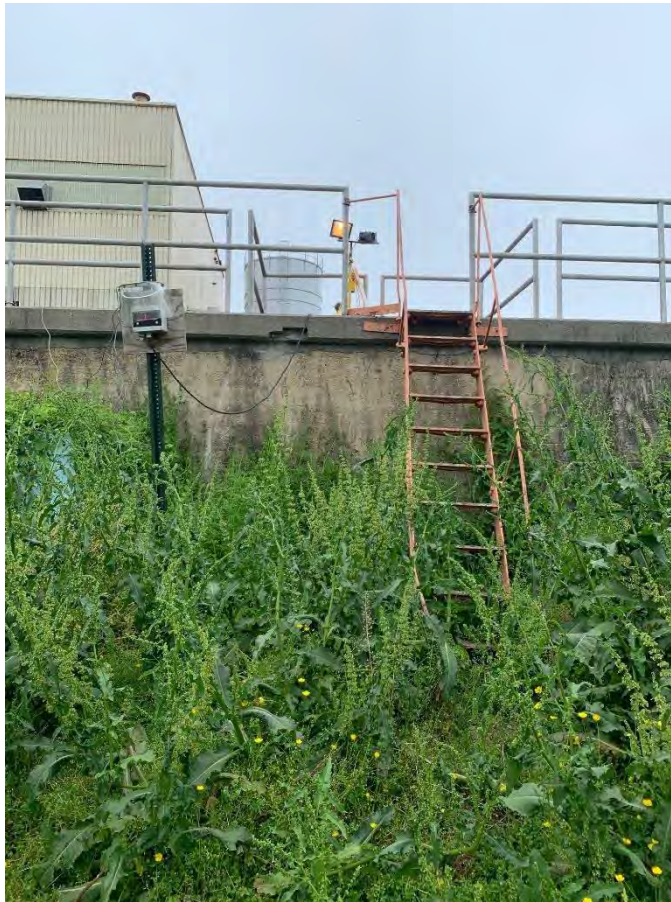
Figure 9 – Sludge Storage Tank 26 with Overgrown Vegetation and Inadequate Lighting
