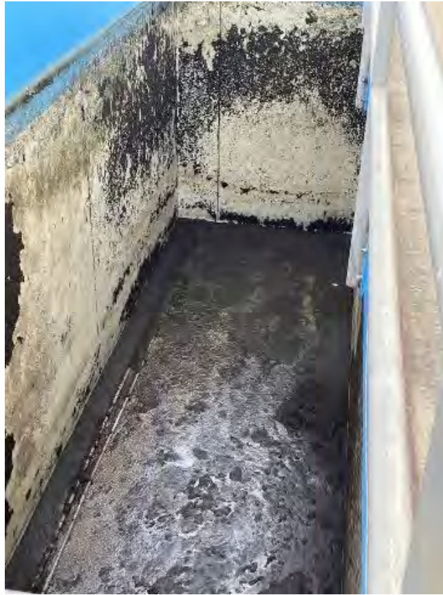
Figure 11 – Drained and cleaned chlorine contact chamber. DPW employees completed entry, unclear if permitted confined space entry procedures were followed.
