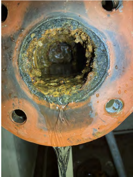
Blower Water Booster Pump #2 – seized potable supply valve
