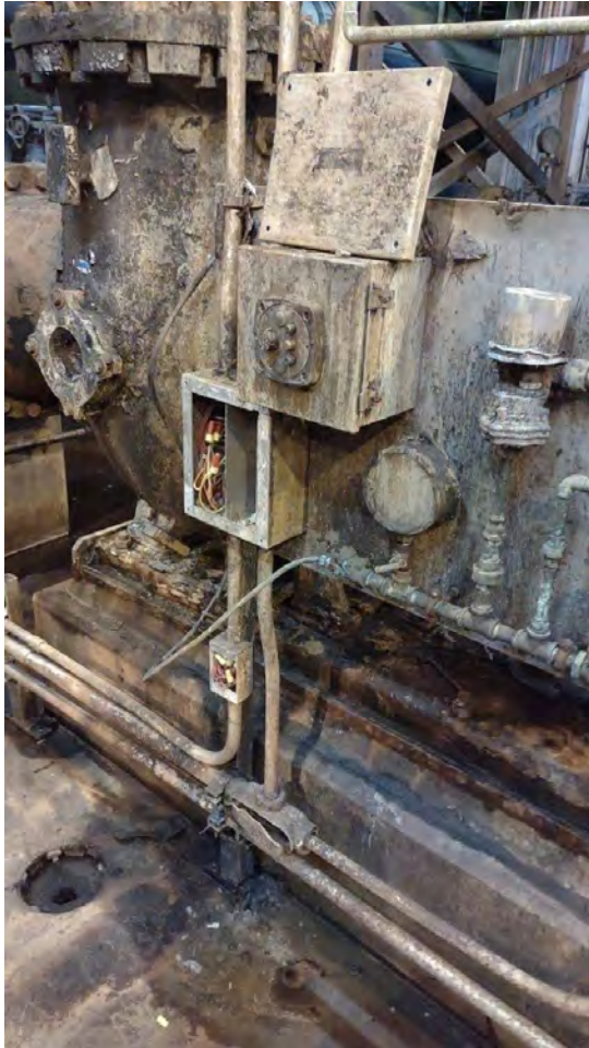
Sludge Pump Bldg. #4 Actuators 14AB, 14B – new wire installed
