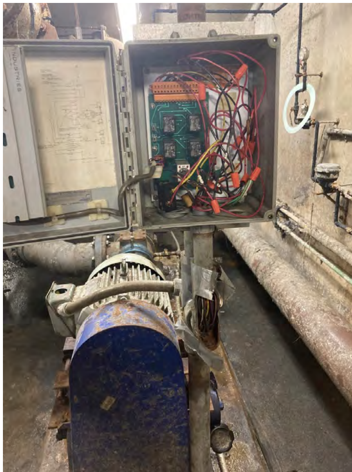
Thickened Sludge Pump 3B – Control Panel & Junction Box with duct tape
