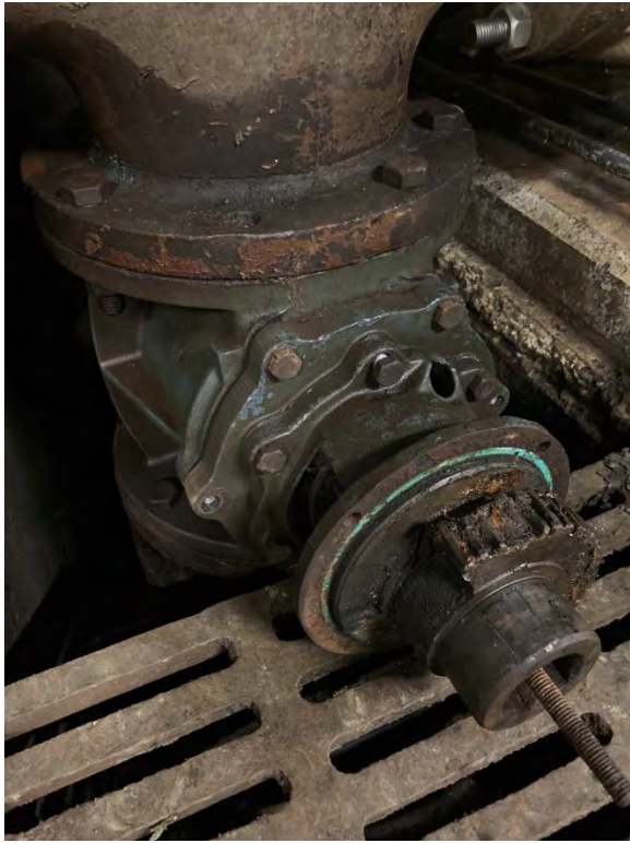
Pump Station #2 RAS – Pump seals to be replaced
