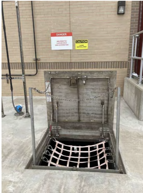
Figure 10 – Apparent Confined Space (Vault)
