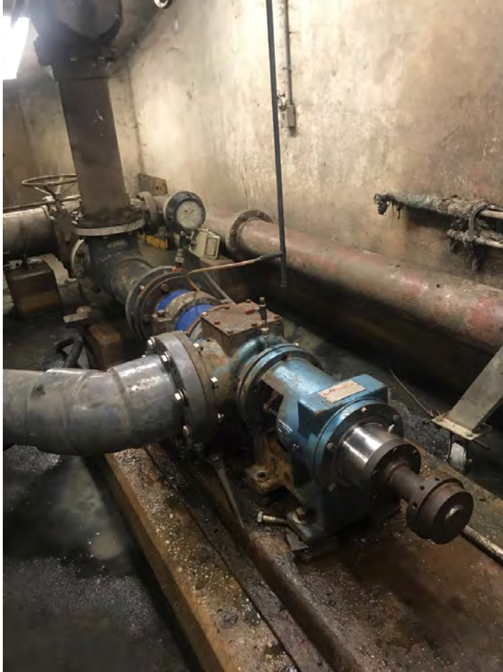
Thickened Sludge Pump 3B Install
