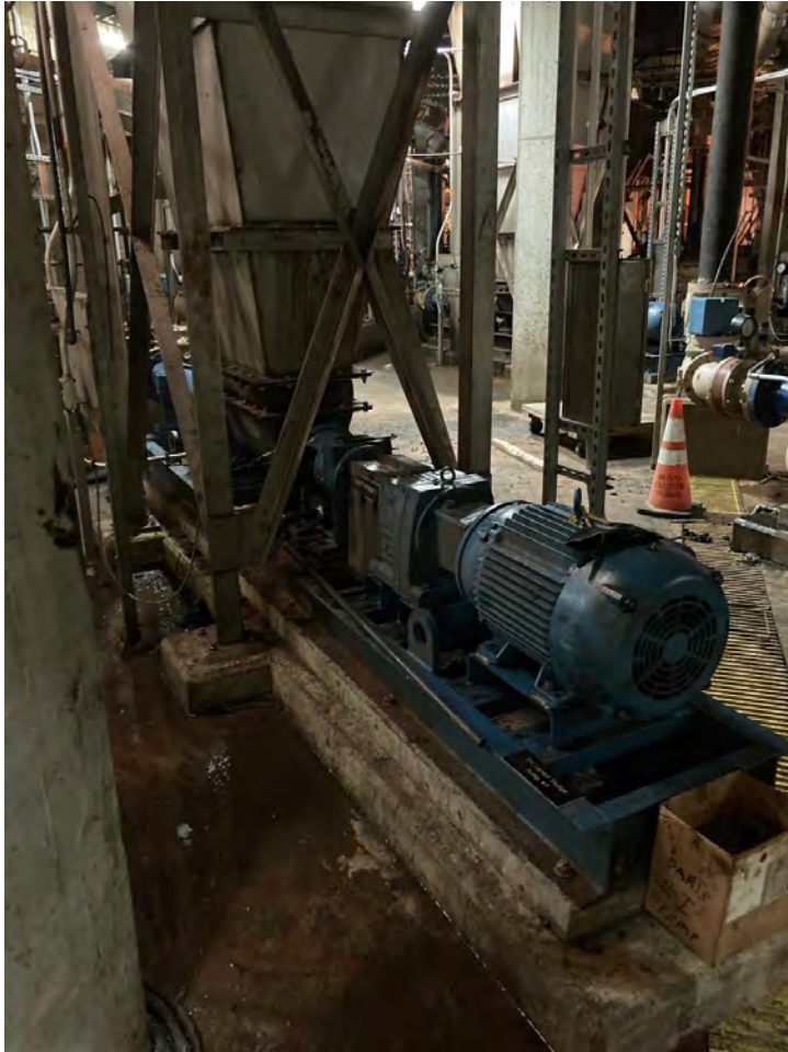
Thickened Sludge Pump #7
