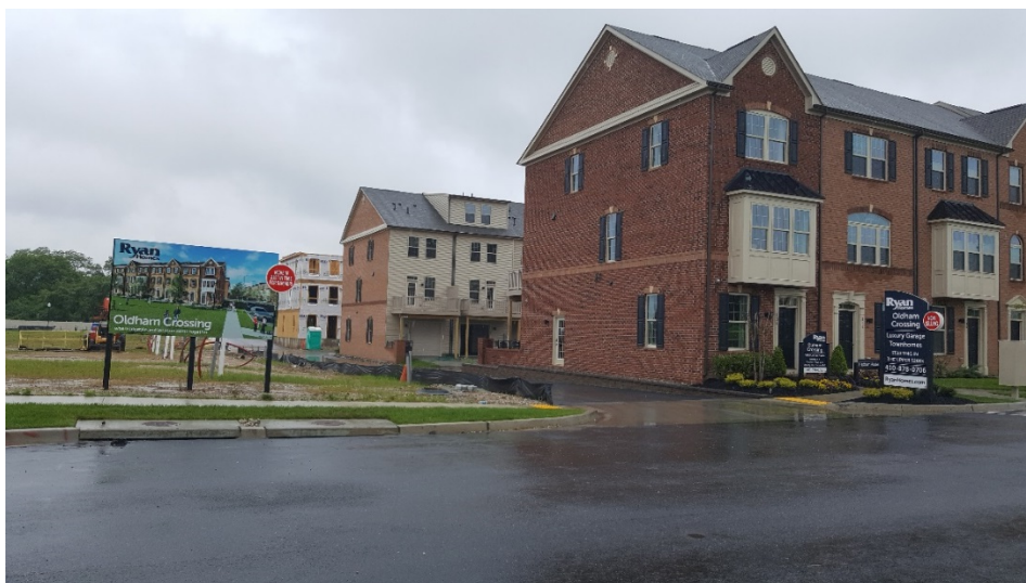
Figure 4: Recent Construction at Oldham Crossing
