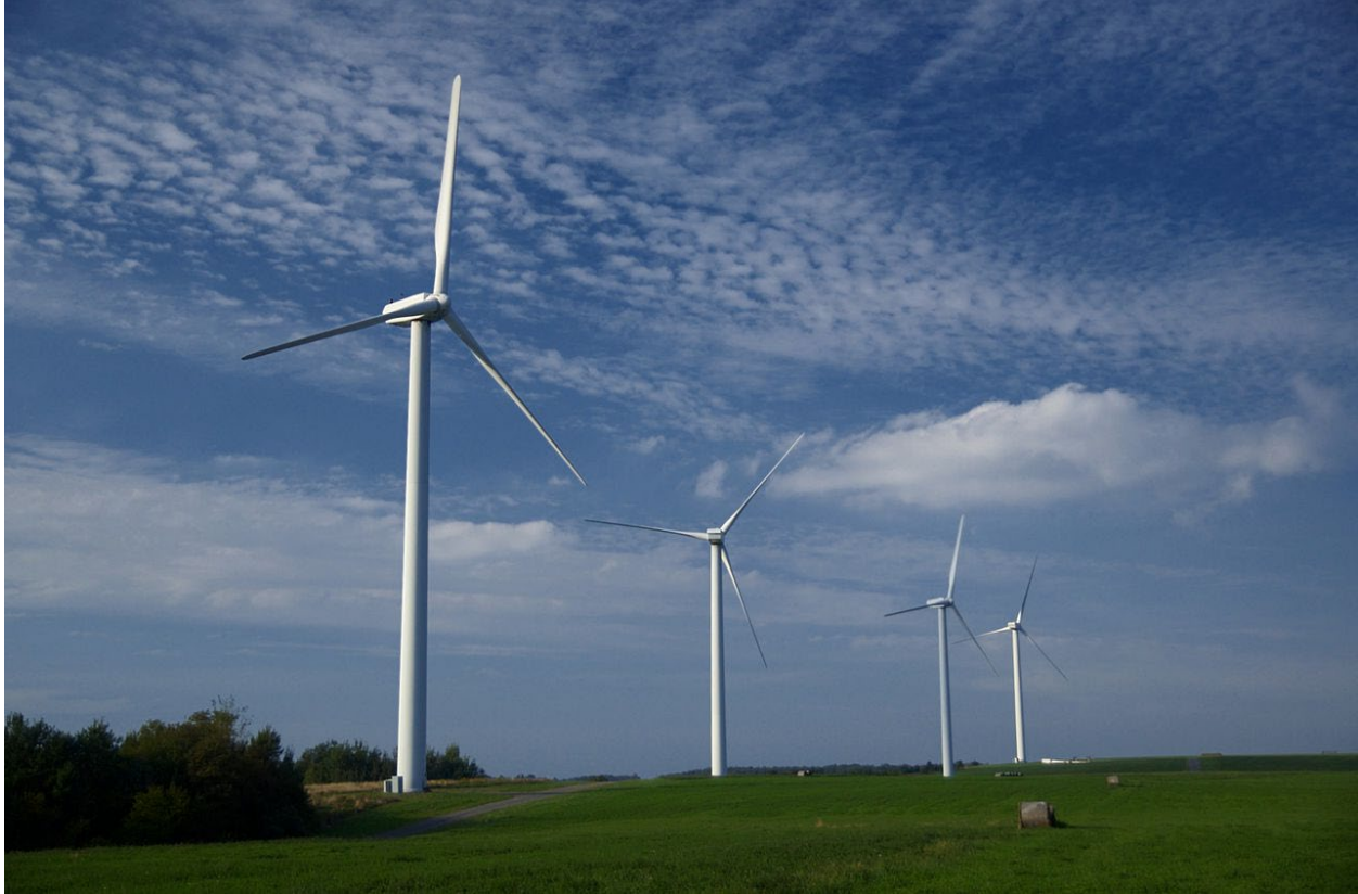
Somerset Wind Farm, Somerset, Pennsylvania Wikimedia Commons; photographer: Jeff Kubina from Columbia, Maryland
