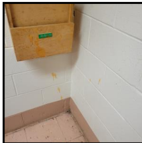
Dining Hall Wall
