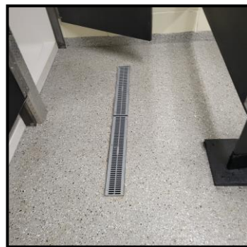
New Drain and Floor
