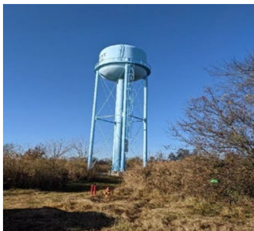
Sandy Point State Park Water Tower
