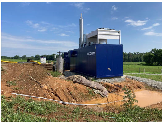
TEDOM Anerobic Digester/Generator at Long Green Farm in Rising Sun, Maryland
