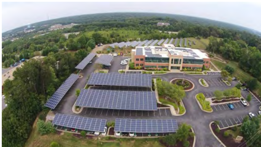
Figure 5 – Aerial View of Solar Installation at MES Headquarters
