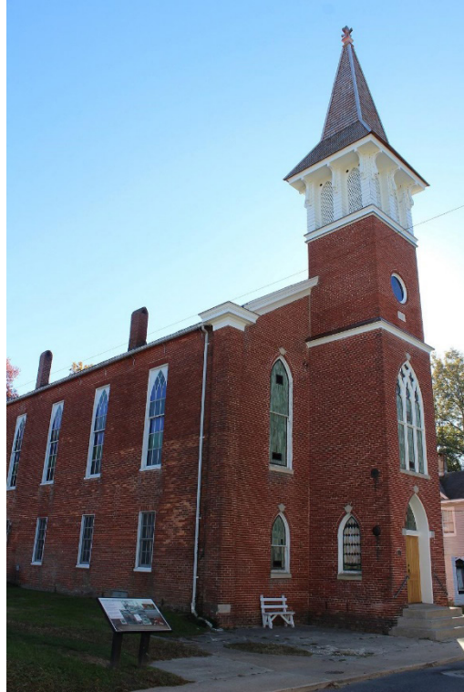
Asbury United Methodist Church, Easton, Talbot County
