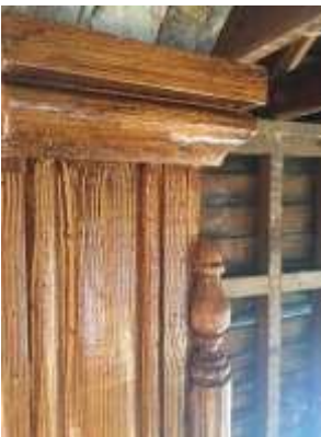
Above left and center: Restoration of the faux grained surfaces. Above right: Careful removal of layers of paint revealed the original treatment to be faux graining.
