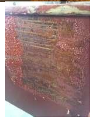
Above left and center: Restoration of the faux grained surfaces. Above right: Careful removal of layers of paint revealed the original treatment to be faux graining.
