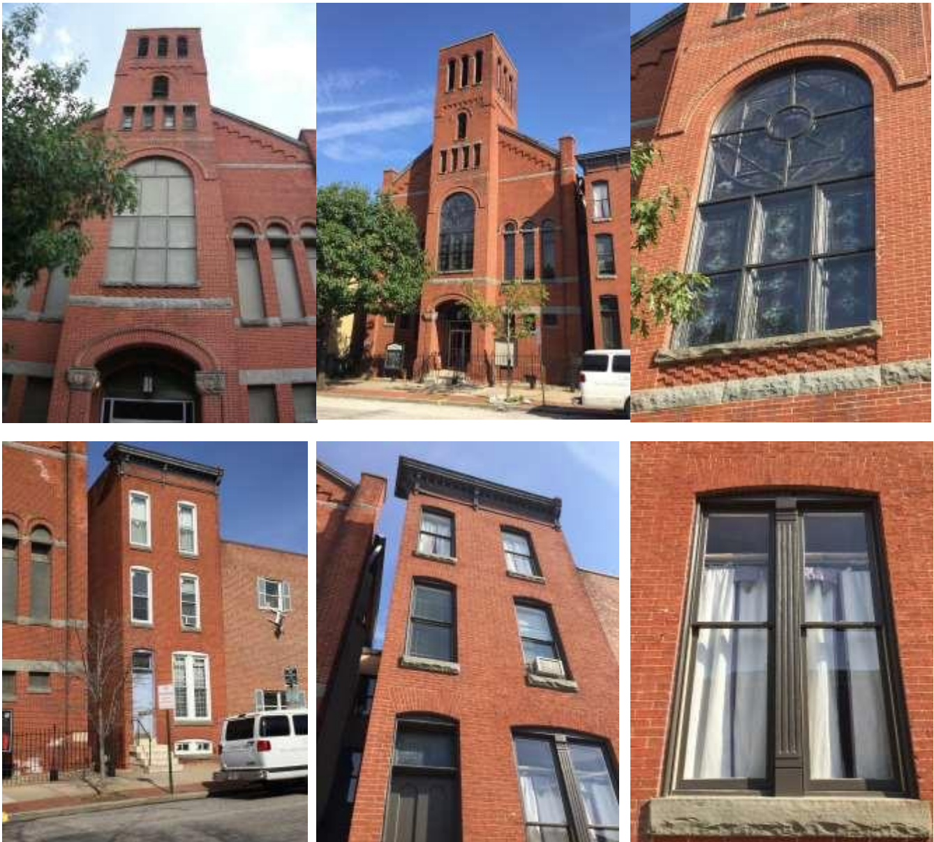
Before, after, and close-up photographs of the church (top) and parish house (bottom).
