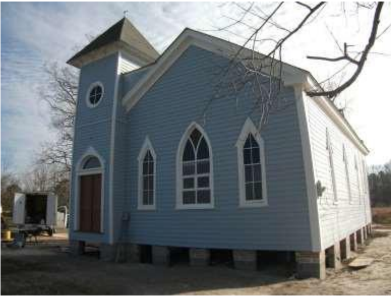
Above: The exterior rehabilitation of the church nears completion.
