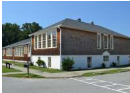
Below: After rehabilitation.
