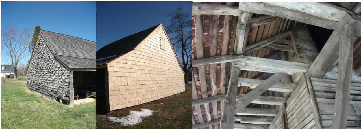
Above left and center: The corn crib's shingles before and after restoration.
