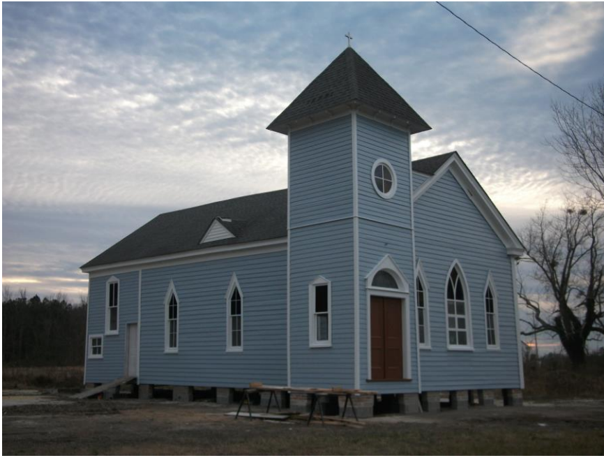
Left: Christ Rock Church after restoration of doors, windows, and siding.
