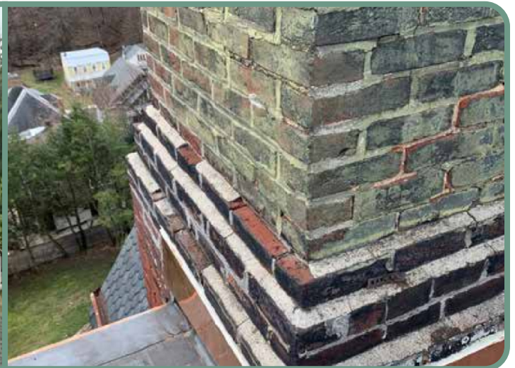
FY24 homeowner project to fix chimney flashing
