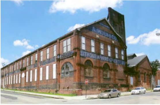
Lion Brothers Company Building , Hollins Street, Baltimore City ($1,044,666.00 in tax credits awarded)
