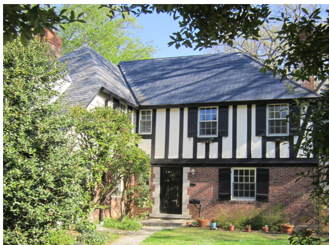
The solar shingles on this Bethesda home are a successful example of clean energy technologies sensitively applied to
