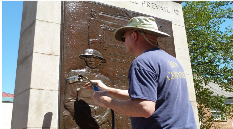
Howard Wellman Conservation applies wax to the Prince George’s County World War I Memorial in Upper Marlboro.
