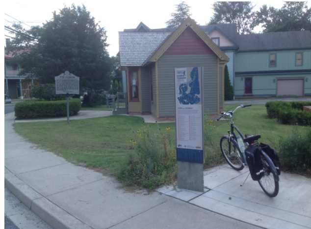
The preservation and restoration of Greensboro's Benjamin House Studio as a museum and visitor information kiosk on the Harriet Tubman Underground Railroad Byway, located in the Stories of the Chesapeake Heritage Area, was supported by Maryland Heritage Areas Authority grant funding.
