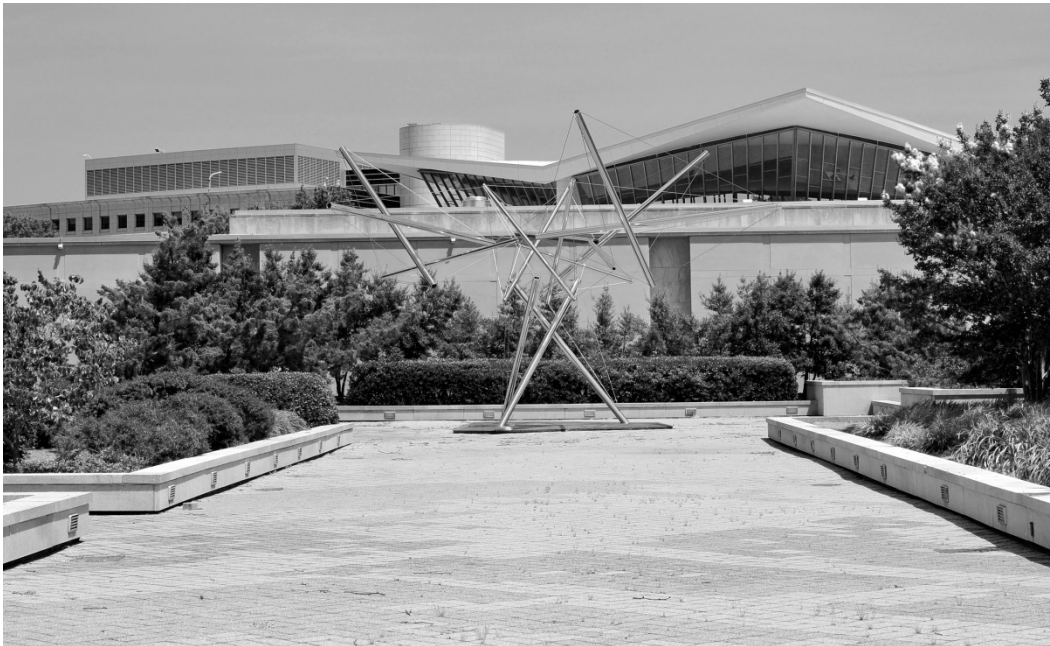
The historic Lister Hill Center and "Tree One" sculpture at NIH's Bethesda campus were included within NIH's survey and documentation of historic properties this year.
