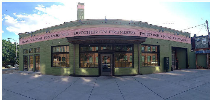
Oak Street Garage, at 2600 N. Howard Street, Baltimore, completed its tax credit supported rehabilitation in 2014.
