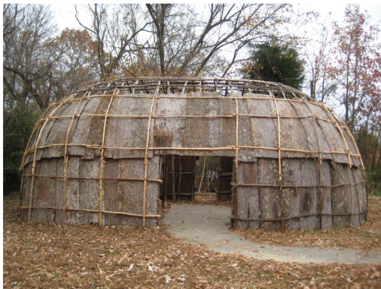
Reconstruction of the Big Lodge, located in the JPPM Indian Village, was undertaken throughout 2013.
