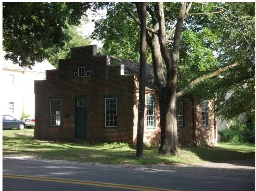
Constructed in 1851, the Uniontown Academy in Carroll County was used as a school and meeting hall central to the small community of Uniontown. Interior and exterior rehabilitation will be assisted through an MHT Capital Grant.
