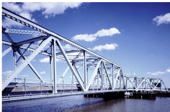
Dover Bridge over the Choptank River is one of Maryland's Preservation Priority Bridges. Built by J.E. Greiner Company in 1932, this three-span steel Warren truss bridge is one of only four remaining historic swing spans in the state.
