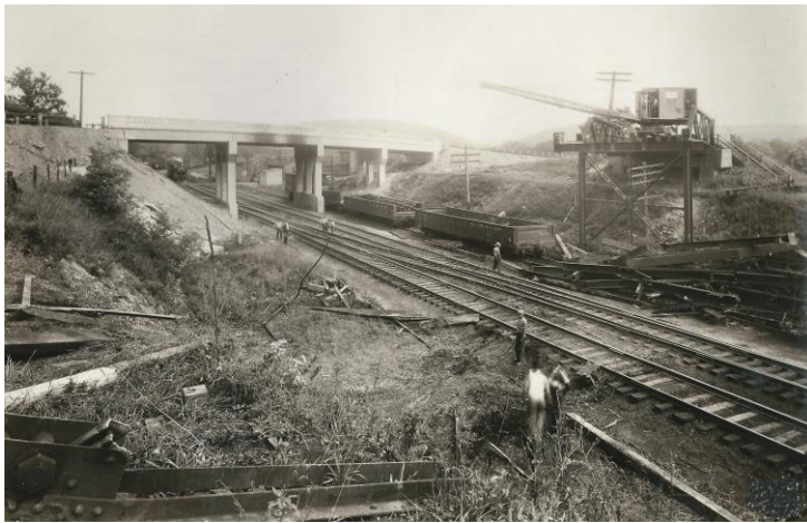
MD 355 Bridge Over CSX under Construction in 1930
