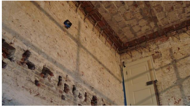
MHT staff helped guide restoration of the Old Senate Chamber.
