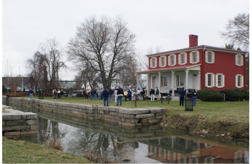
The Lock House, c. 1839, at the southern terminus of the Susquehanna & Tidewater Canal, is a centerpiece of the Susquehanna Museum of Havre de Grace. In 2013, the Maryland Heritage Areas Authority provided funding for repair and repainting of deteriorated second-floor windows and shutters.
