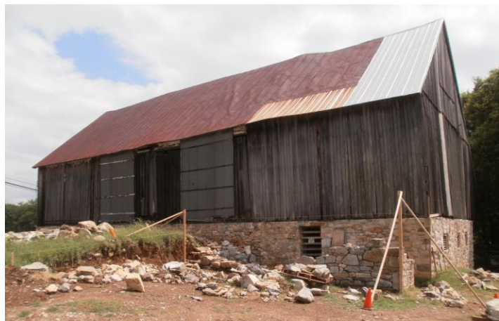
Stabilization efforts at the Newcomer Barn, Antietam National Battlefield
