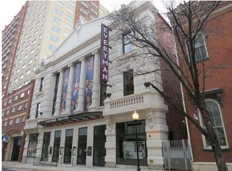
Town Theatre (Everyman Theater), located at 315 W. Fayette Street in Baltimore City, completed its tax credit supported rehabilitation in 2013.
