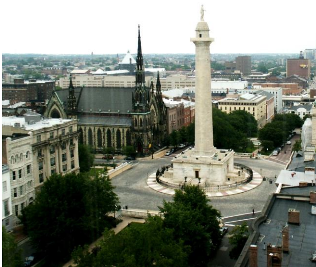
The Washington Monument at Mt. Vernon Square received Maryland Heritage Areas Authority funding for repointing. This project, part of a comprehensive restoration, began in 2013.
