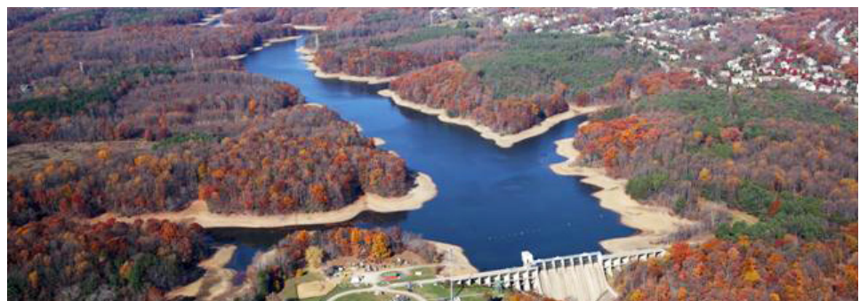
Washington Suburban Sanitary Commission’s T. Howard Duckett Dam on Rocky Gorge Reservoir, Howard and Prince George’s Counties
