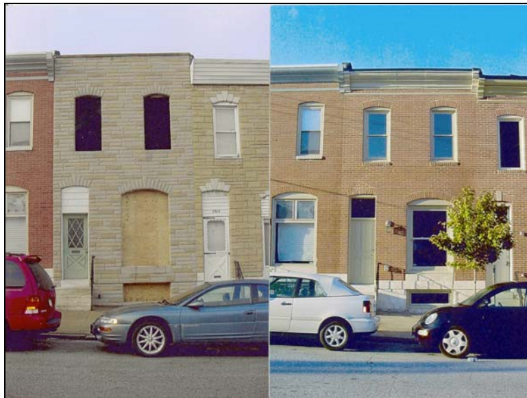
2602 E. Fairmount Avenue in the Patterson Park National Register Historic District in Baltimore before (left) and after (right) a historic property rehabilitation tax credit project. This is typical of small-scale rehabilitation projects.
