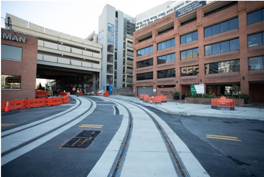
Purple Line track installation at Silver Spring Library (October 21, 2025)
