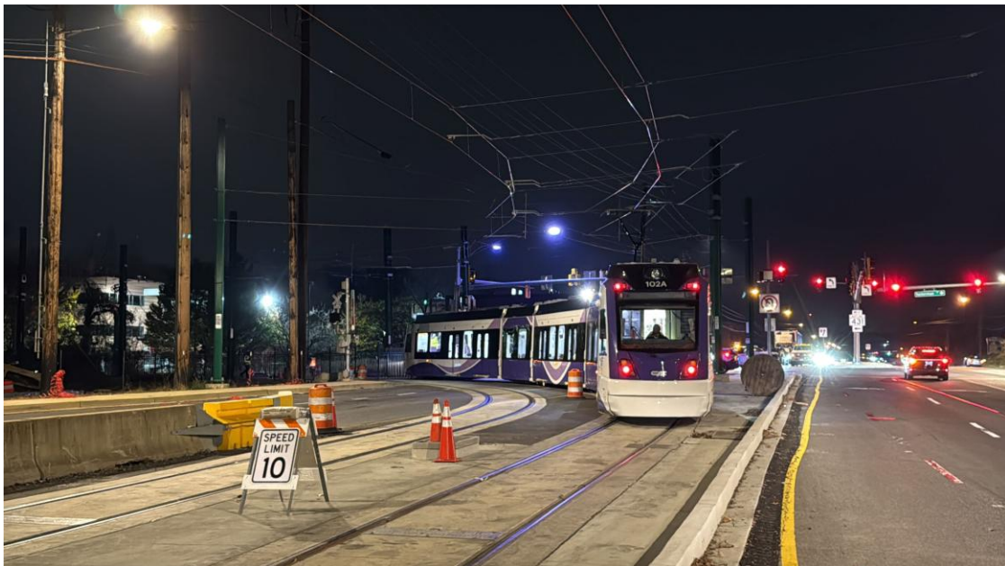
Seg 7 Testing - Site View of the Light Rail Vehicle No. 102A turning onto Kenilworth Ave. (11.20.25)
