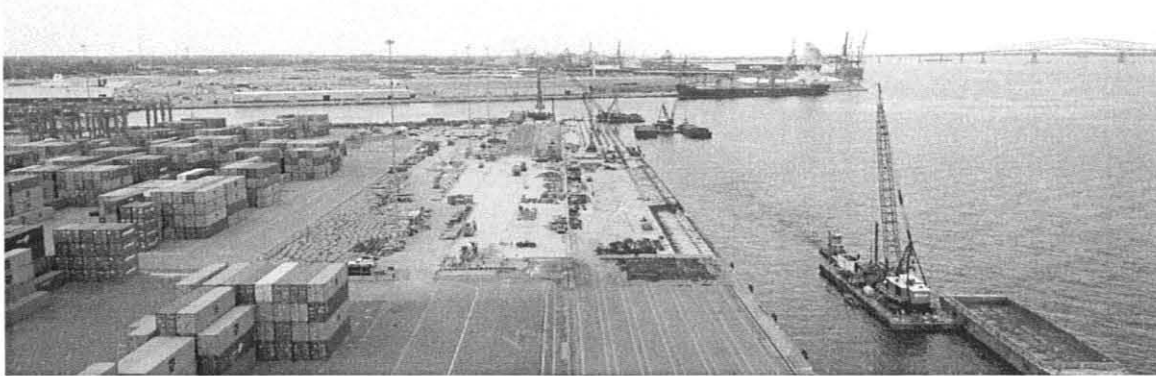
Construction of 50-foot deep berth at Seagirt is underway.
