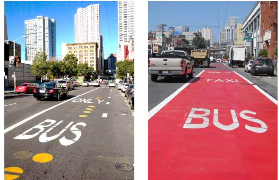
FIGURE 11 SAN FRANCISCO 3RD STREET TRANSIT-ONLY LANE BEFORE AND AFTER RED TREATMENT AND CORRESPONDING VIOLATIONS PER HOUR ALONG THE CORRIDOR
