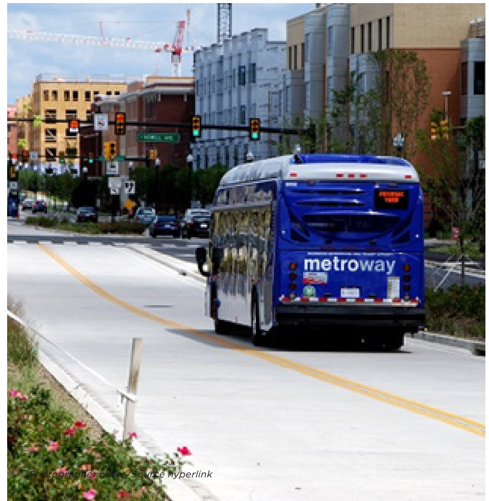
FIGURE 5 MEDIAN RUNNING PORTION OF THE CRYSTAL CITY POTOMAC YARD TRANSITWAY
