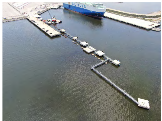
Figure 13 Fairfield Marine Terminal Pier 4, May 2025
