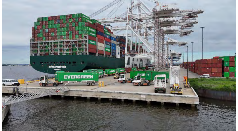
Figure 9 Seagirt Marine Terminal
