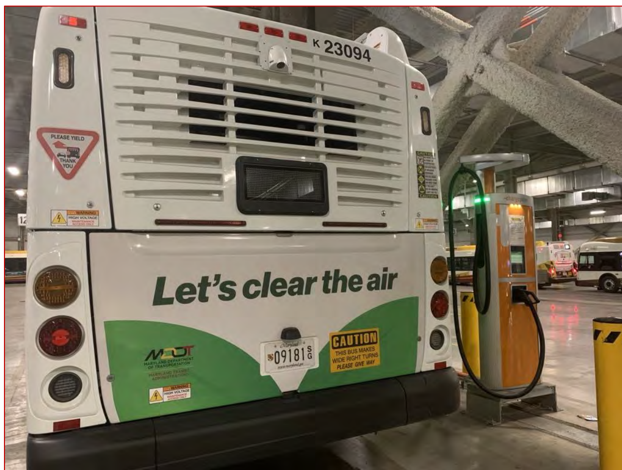
MTA Zero-emission Bus Charging
