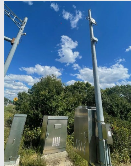
US 1 & MD 100 DSRC/ C-V2X RSU/OD Sensor.
