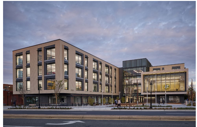
College Park City Hall in College Park, Maryland earned LEED Gold in 2024
