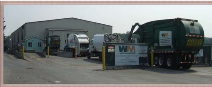
The largest processing and transferring facility in operation, Annapolis Junction Transfer Station, Jessup
