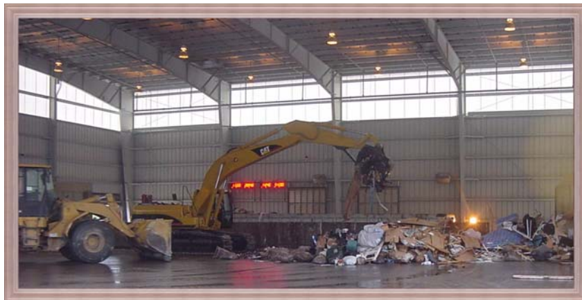
Processing Facility and Transfer Station.
