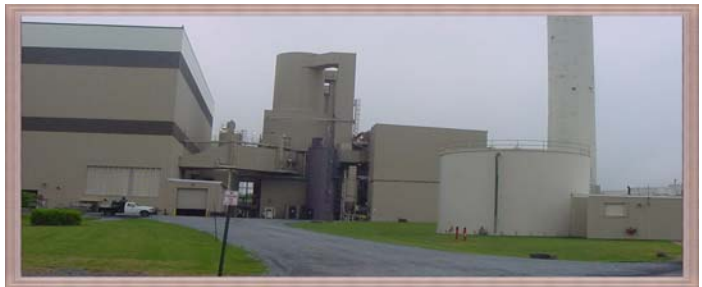
Waste-to-Energy facility at Dickerson, Montgomery County
