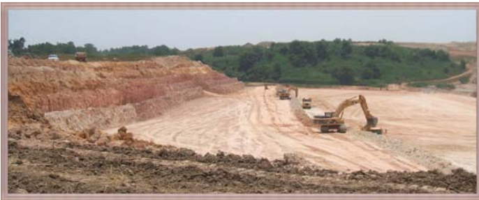
New cell under construction at Quarantine Road Landfill, Baltimore City
