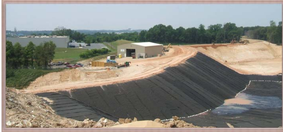
Rubble Landfill Liner Installation.
