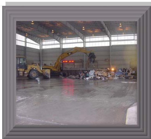
Alpha Ridge Processing Facility and Transfer Station (Opened in 2005).
