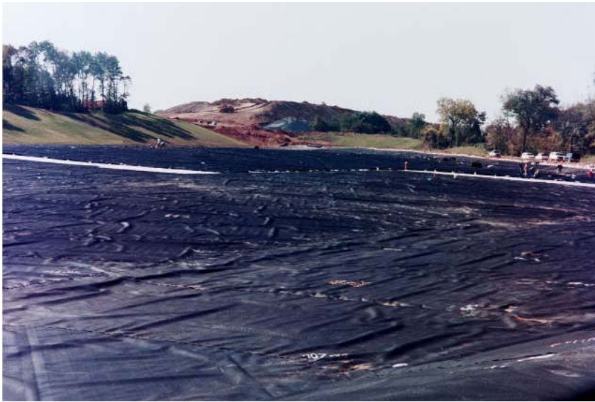
Picture 3. Landfill liners prevent the release of contaminants and help protect groundwater when properly designed and constructed. MDE scientists and engineers review plans and inspect construction quality assurance for municipal, industrial, and rubble landfills in Maryland.
