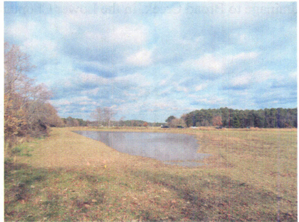
Russell Train Site Area #3 after grading
