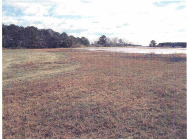
Russell Train Site Area #3 after grading
