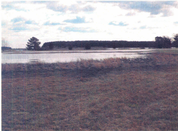
Russell Train Site Area #3 after grading
