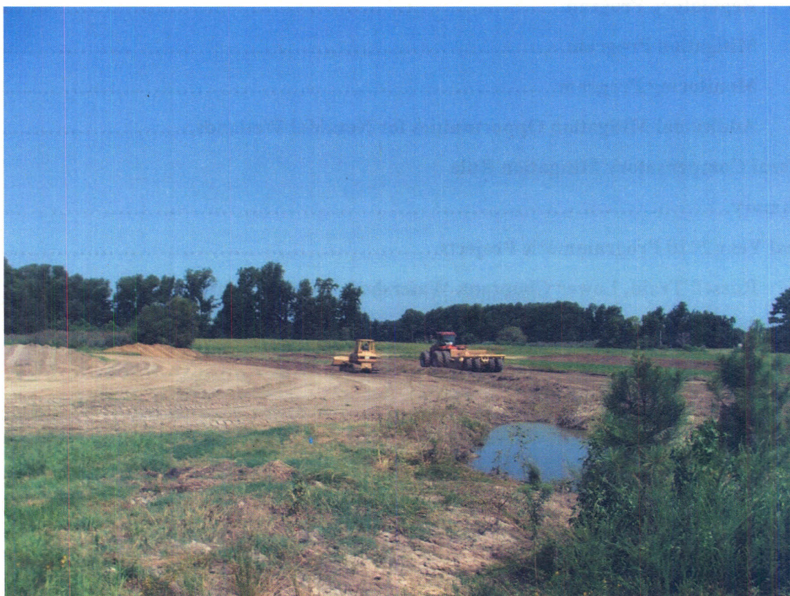
Russell Train Site during Construction
