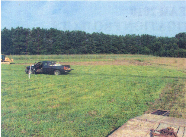
Russell Train Site during construction
