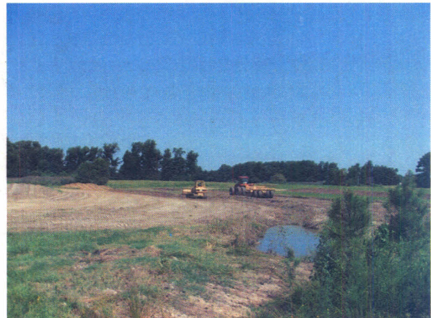
Russell Train Site during construction
