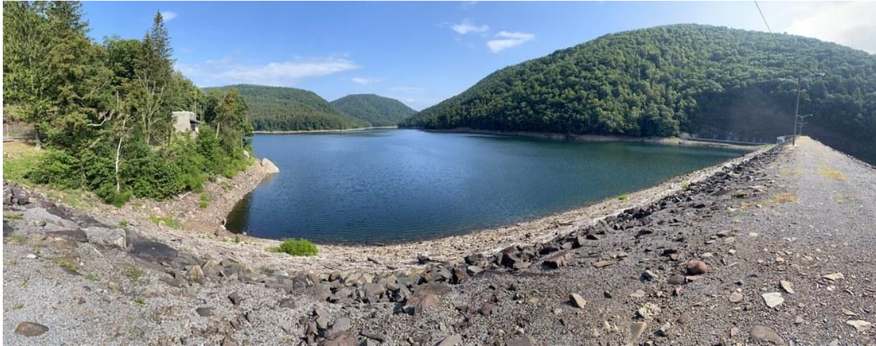
Savage River Dam, Garrett County Maryland
