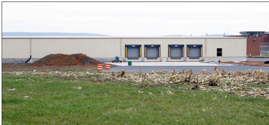
New Addition to Hagerstown Warehouse is Completed
