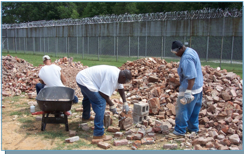
MHC Deconstruction Project
