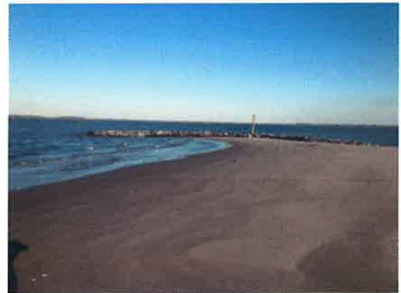
Dredged sand from Kent Narrows was used to replenish the shoreline at Ferry Point Park. Native grasses have since been planted to stabilize the site. Photo credit: Maryland DNR
