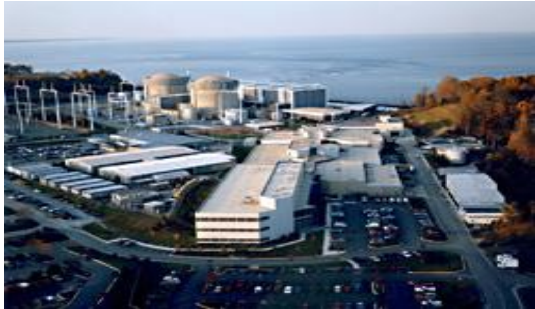
Figure 1-1 Calvert Cliffs Nuclear Power Plant
