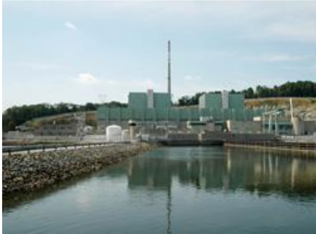
Figure 1-2 Peach Bottom Atomic Power Station
