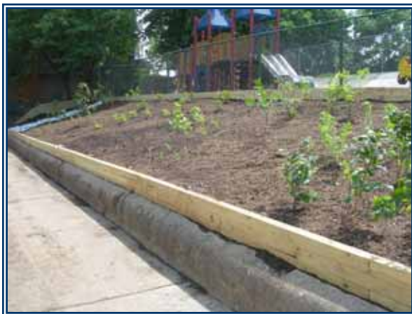
Impervious surface removal and native vegetation planting at North Mount Street.
