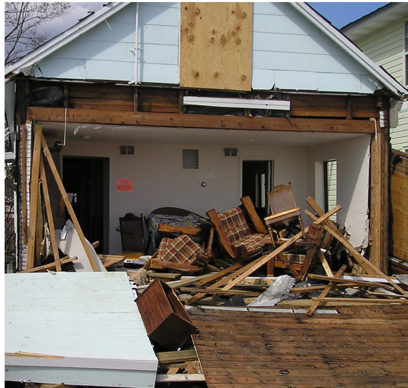
Damage from Hurricane Isabel
