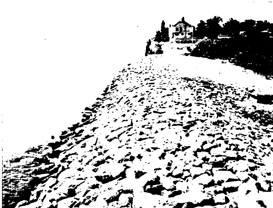
Town of Chesapeake Beach, Shore Erosion Project, southern half of stone revetment and back-drop
