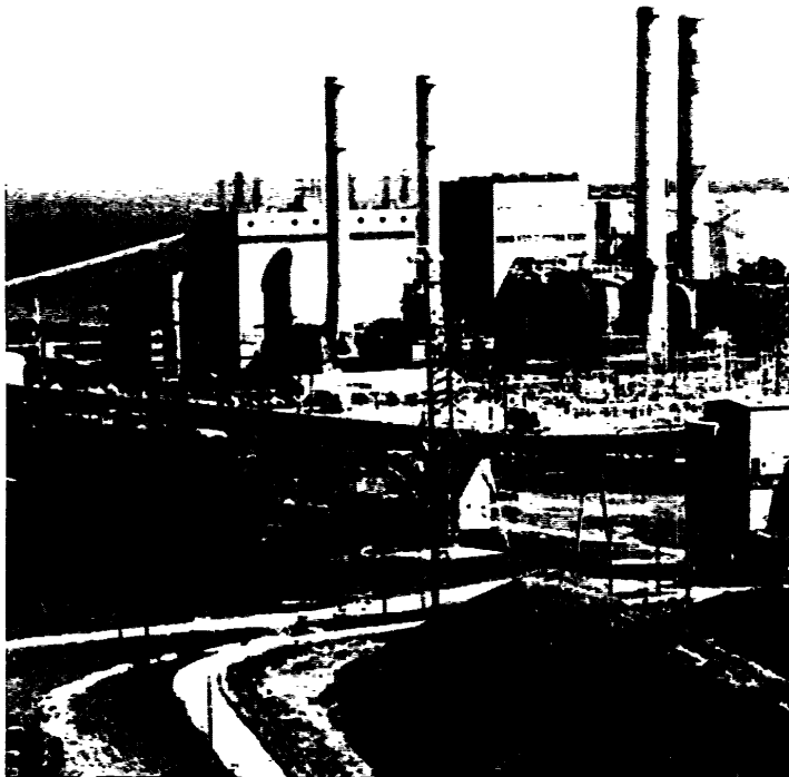
Maryland Power Plant
