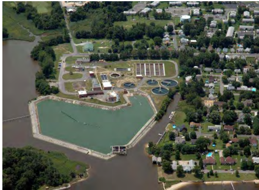
Cambridge Maryland, Wastewater Treatment Plant
